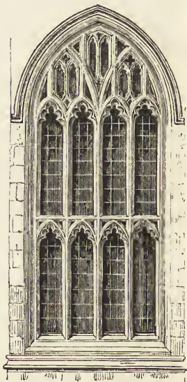
150. New College, Oxford, A.D. 1386. Shewing Perpendicular tracery, with sub-arches and a transom, the heads of the lights cinquefoiled.
